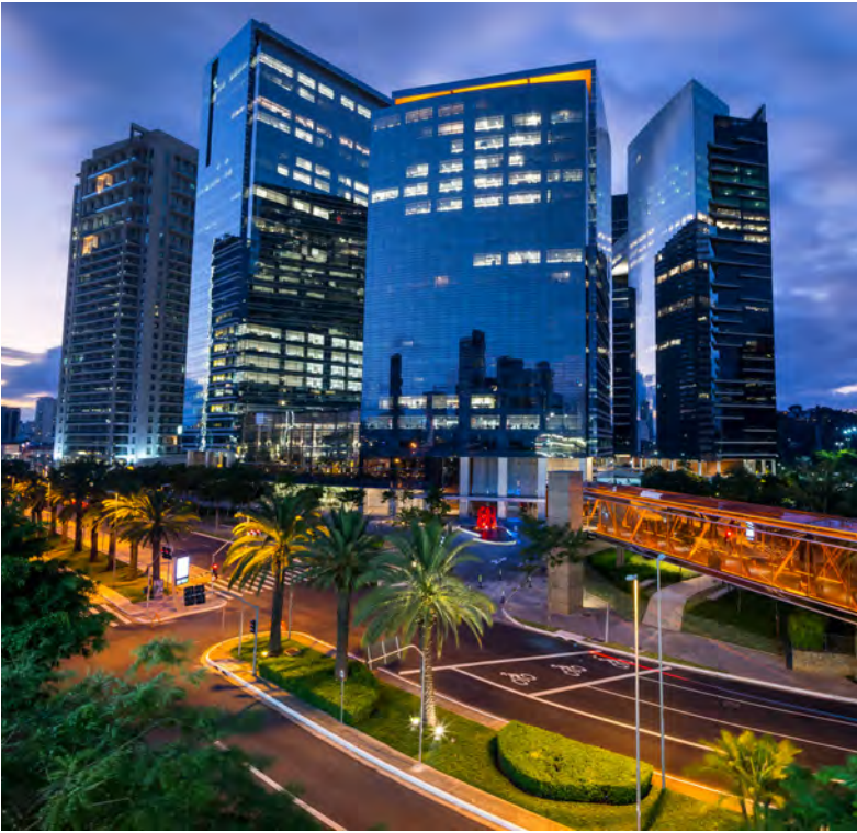
Multiplan’s Morumbi Corporate Towers, comprised of more than 700,000 sf. of AAA LEED Gold leasing office space in São Paulo, Brazil.
