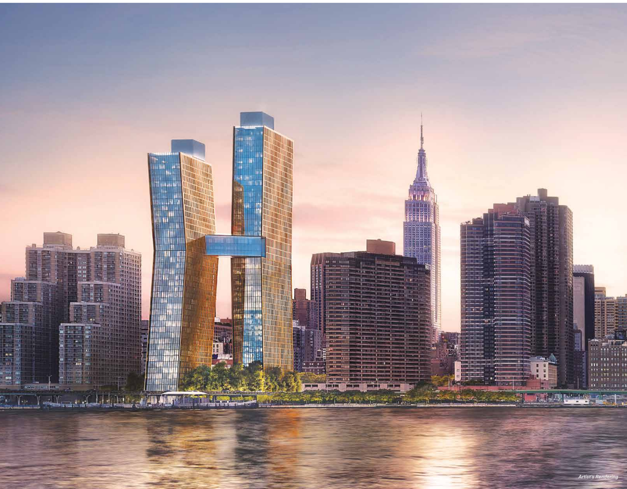
American Copper Buildings / New York
